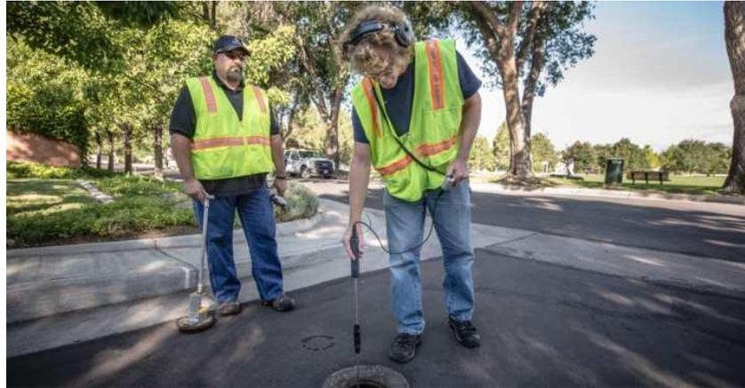
*Detection of leakage by sounding rod method*
