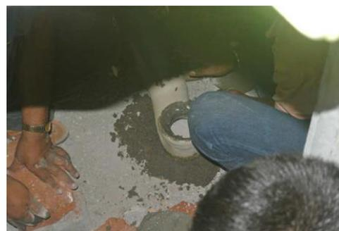
P-trap. Now place the P-trap on it by jointing its discharge end with the soil pipe. Thoroughly support the P-trap.
